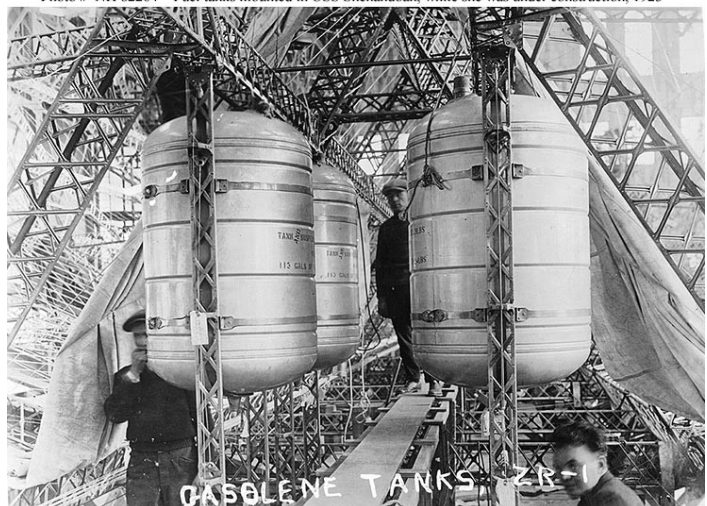
Photo # NH 82264 Fuel tanks mounted in USS Shenandoah, while she was under construction, 1923
